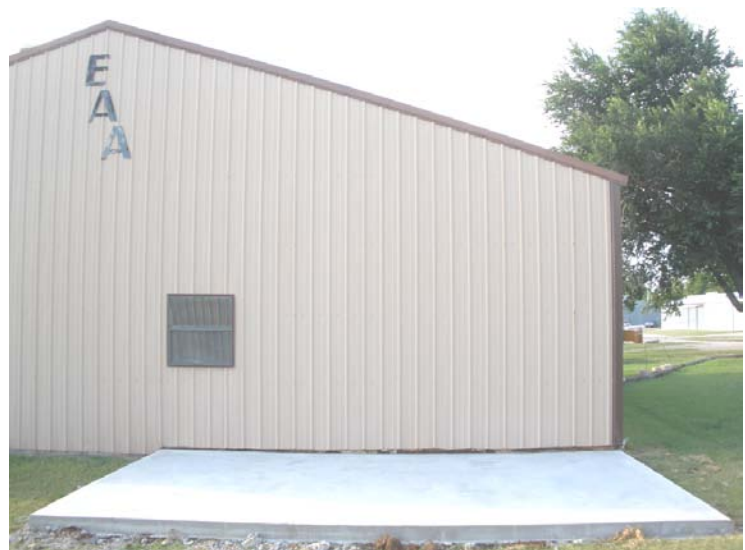
Concrete slab poured for new storage area.
